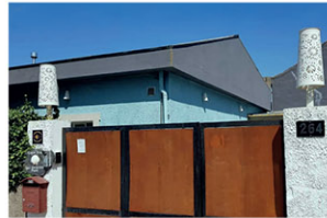
Albergue de Peregrinos Via Portus Cale International Association | Via Portus Cale International Association Pilgrim's Hostel – Matosinhos
